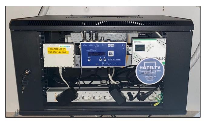
Before disconnecting the Telekom power supply, its signal level was measured and set 3 dB higher than the measured value at the Ekselans Eksel amplifier output. Thanks to the change of modulation (DVB-C instead of DVB-T) and the higher initial signal level, reception was perfect even at the furthest reception points, although there had been many complaints of fringing before.
